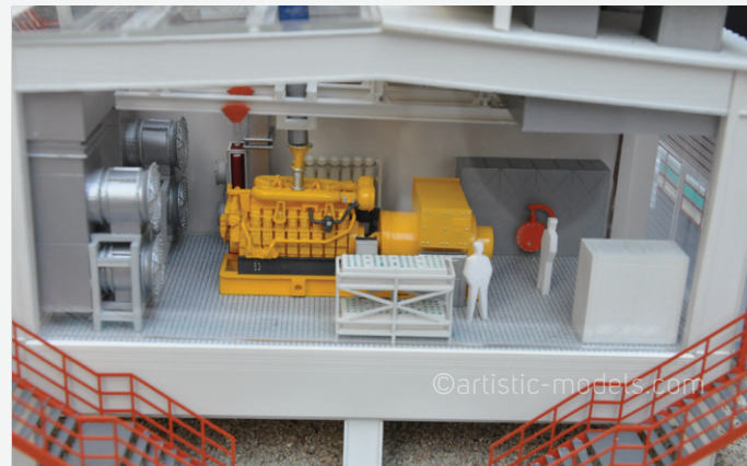
Emergency Diesel Generator Skema
